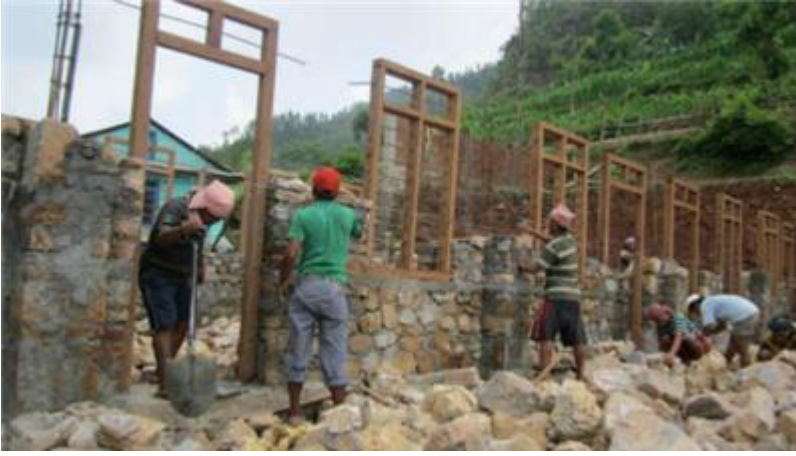
Construction of the ground floor.
