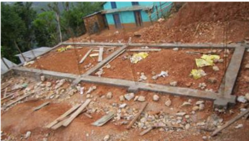
The foundation of the new building.
