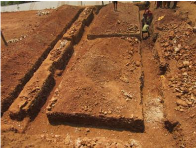
Excavation of the trench for the foundation.
